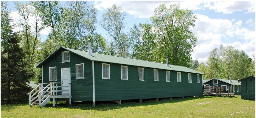
Restored building at Rabideau CCC camp in Minnesota
