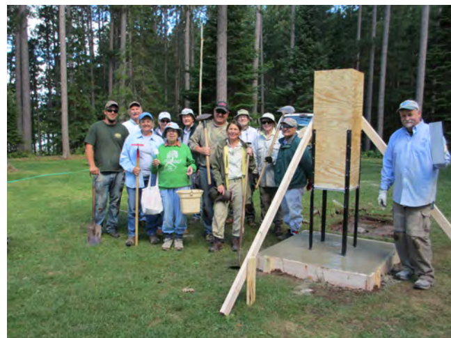
Crew for the foundation work
