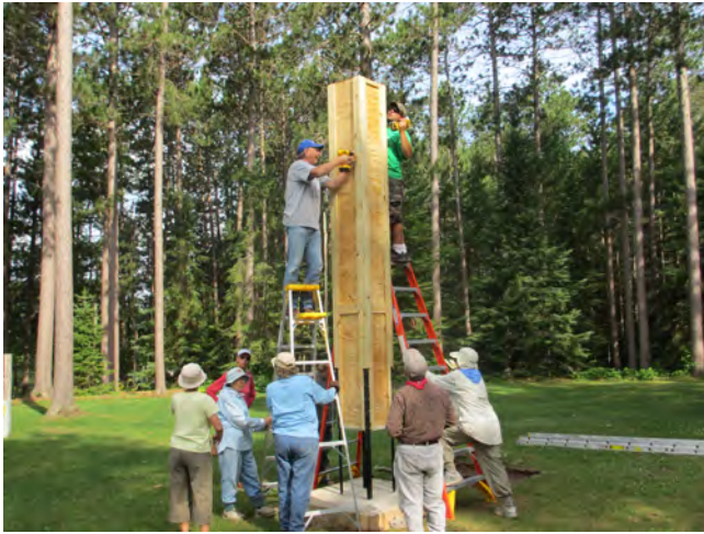
Ladder-work was required for the 12' tower.
